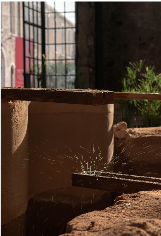
Fig. 5. Channels of condensate water directed towards landscapes.
